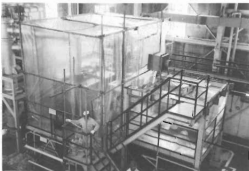
Photo 1 Greenhouse of Furnace
