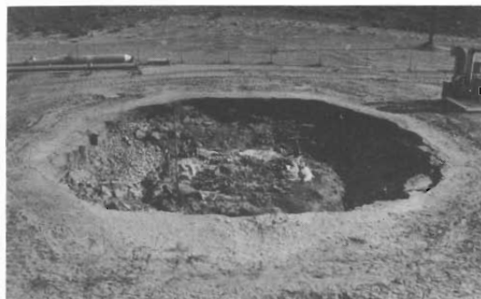
Photo 1 Depression Due To Volume Reduction (About 10m Diameter)
