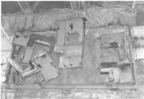
Photo 2 Dismantling of Furnace
